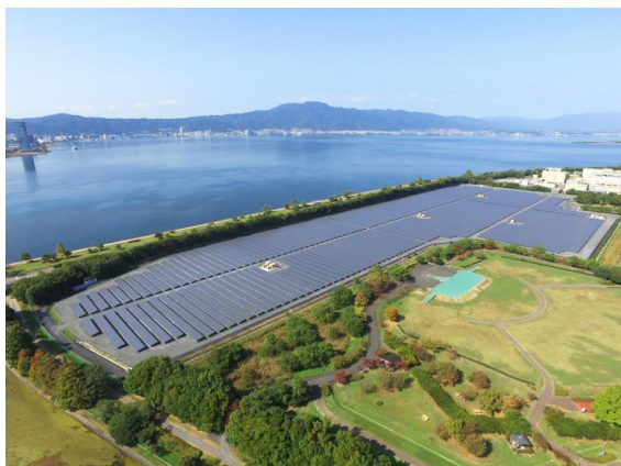
8.5 MW mega-solar power plant on Yabasekihanto Island
